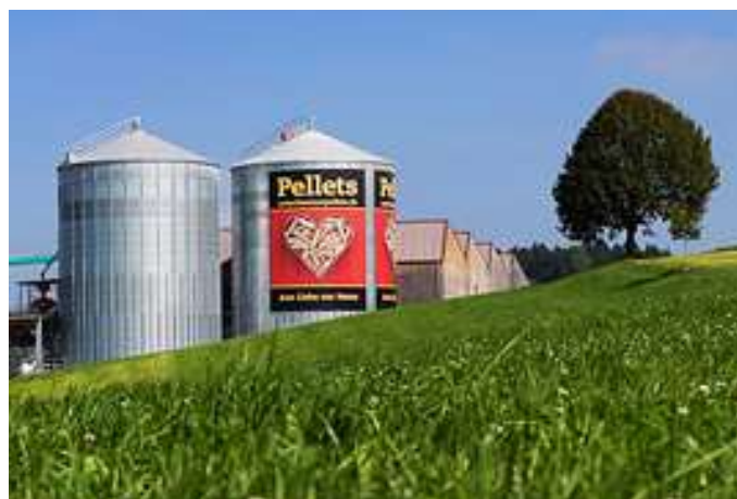
Figure 6: Pellet silo of 2200 tons capacity ( www.ostschweizerpellets.ch )
